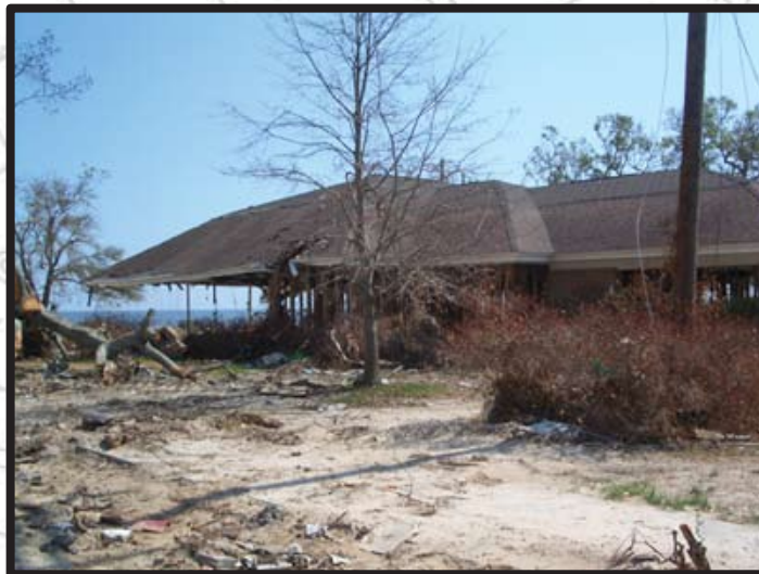
Our Lady of the Gulf Parrish Rectory Destroyed Barter & Associates is Designing a Replacement
