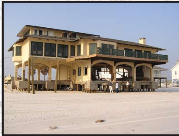
Company Engineers Inspect Residence in Gulf Shores
